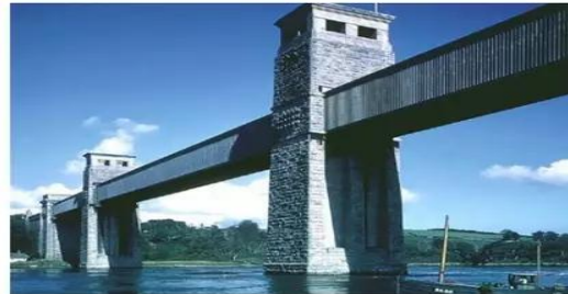
Britannia Tubular Bridge ↔ Wrought Iron
